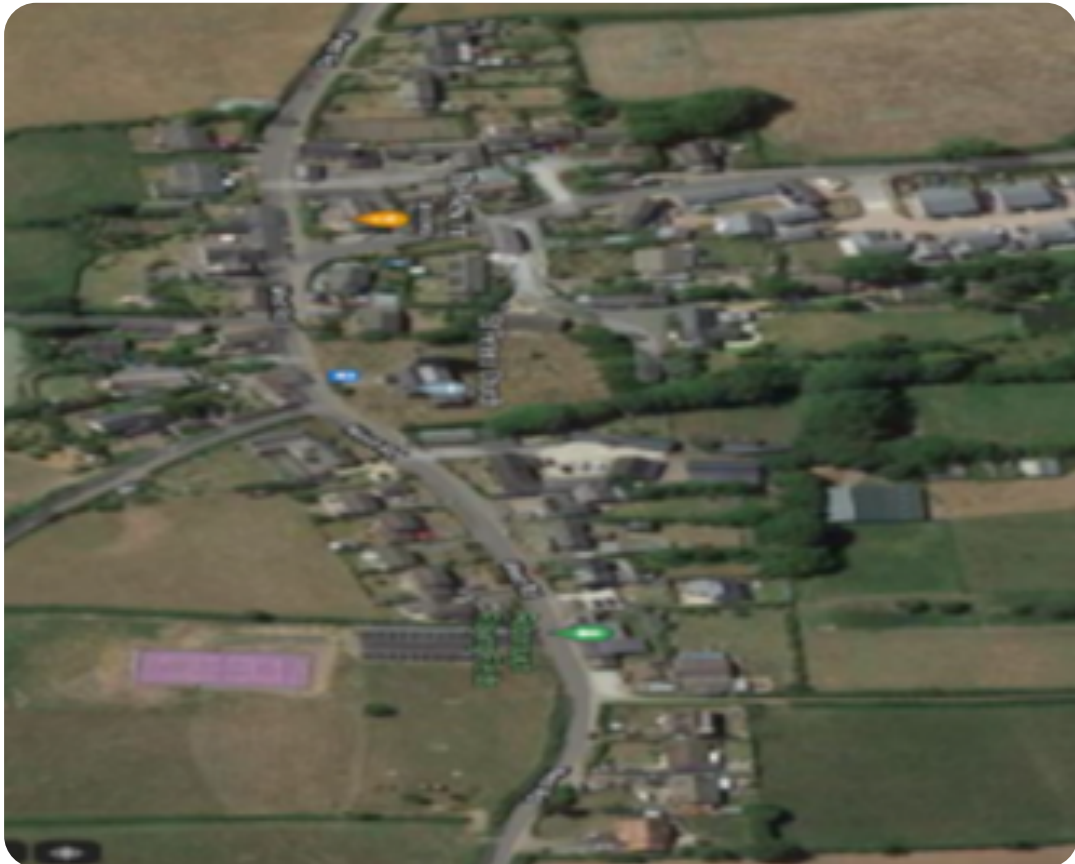
Image: Roborough (reproduced with permission from Homes England)
